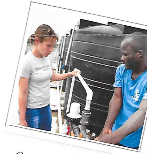
Emily installing a chlorinator at a clinic.
